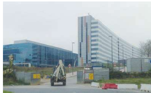
Oviedo Central University Hospital (Asturias/ SPAIN) The air conditioning ducts are constructed with URSA AIR: M2021 Aluminum Roll.
