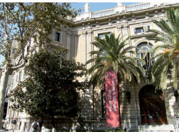
Lawyers College of Barcelona. Ducts were done with URSA AIR AI-TECH2.
