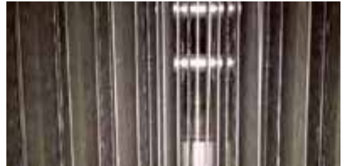
Uneven spacing of ion plates
