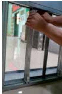
Install the upper buckle
