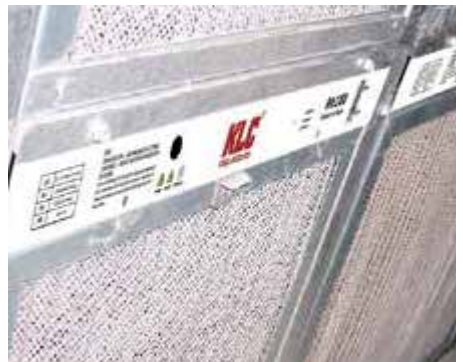
Seal the gaps between the mounting frames with sealant
