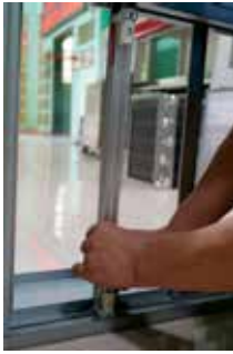
Remove the lower light buckle
